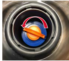
Turn Filters Counterclockwise to Remove
